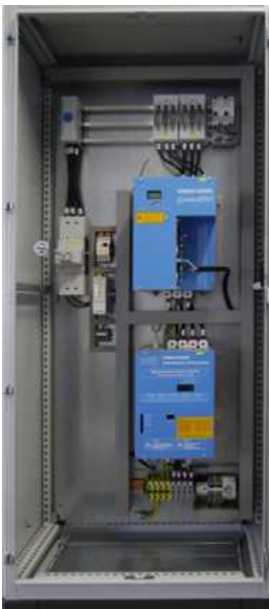
Fig. 8-1 Control cabinet with GeniusHWI master/slave
